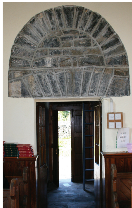
Earlier doorway with double arch
